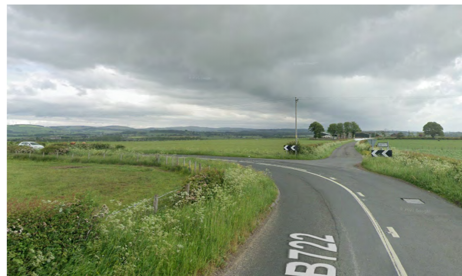
Breaconbeds bend between the site and the A74(M) may require improvement to address issues of visibility and road safety for HGVs.
