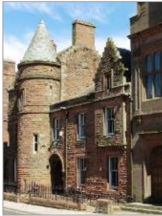
former Police Office
