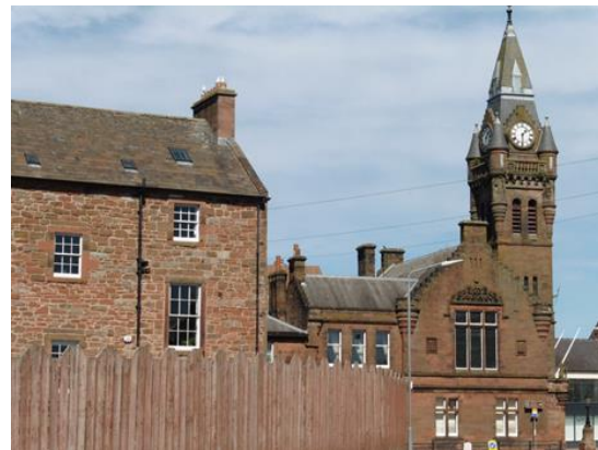
Rear of Bridge House
