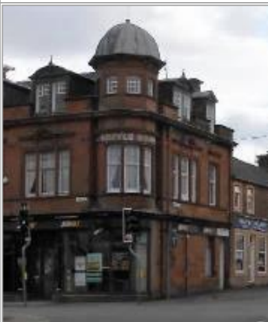
Argyle House 121 High Street
