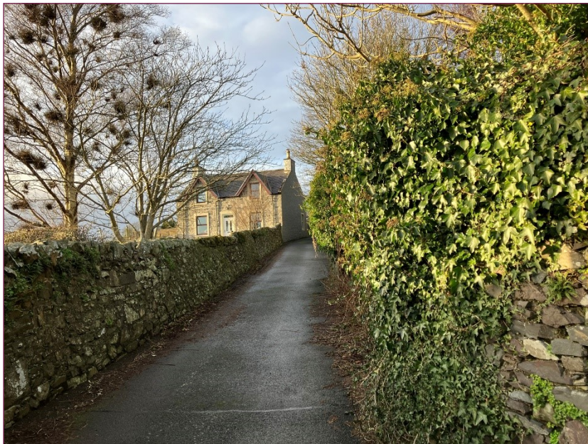
Top: Looking north up Kilquhirm Road at the whinstone boundary walls;
