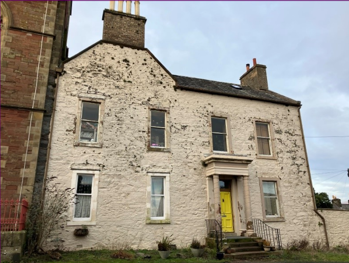
Fairholme, South Main Street was built early in the 19th century as a bank house originally facing south-west but when County Buildings were built, a new side entrance was made with a Classical Doric style door piece.
