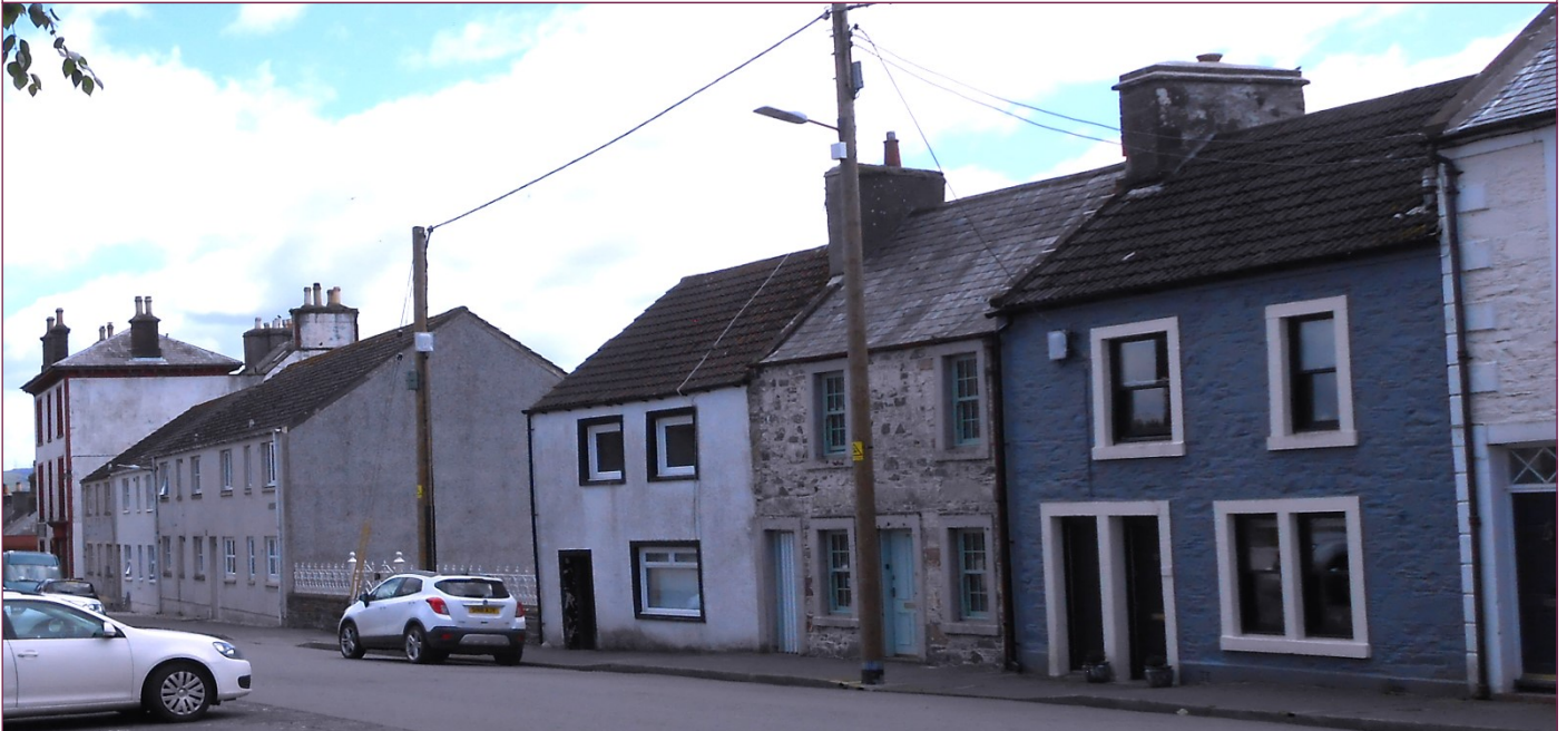
Above: Northern part of South Main Street with a mix of bare stone, smooth rendered and painted, 2-storey, 3-bay buildings and a modern grey rendered terrace.
