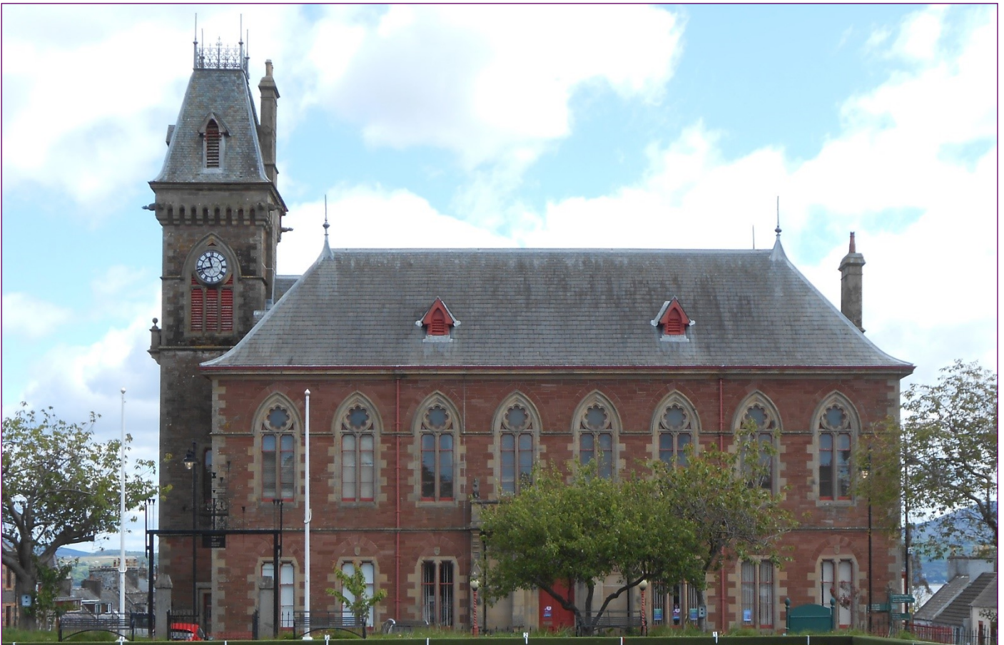
B Listed Wigtown Town Hall and Library, built as the Sheriff Court in the 1860s; designed by Thomas Brown II. The tower includes part of a 1756 building. The red sandstone building with buff sandstone dressing in 'French Gothic' style. It faces west-south-west, dominating the eastern end of the Market Place and recreational space.
