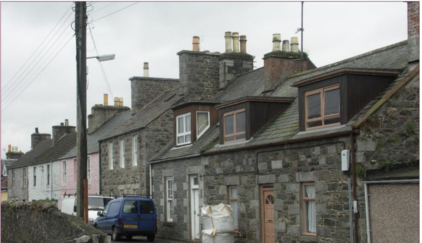
Above: Traditional dwellings on Lochancroft Lane of mixed designs. The large chimneys are significant in the roofscape and the majority of the elevations are whinstone and granite, some painted. The dormers are later additions and do not have traditional shapes or material finishes. Doors and windows are a mix of modern and traditional formats.
