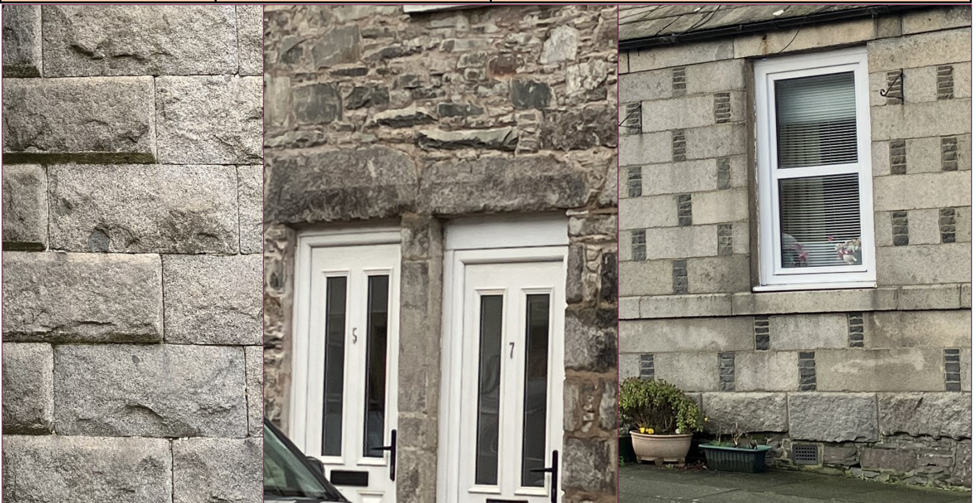
Left:- Coursed, rough faced, cut granite blocks in an elevation; Middle:- roughly hewn, granite lintels above paired doors; Right:- coursed, plain, granite blocks with mouse ladder whinstone snecking between and a granite string course and granite block footings.
