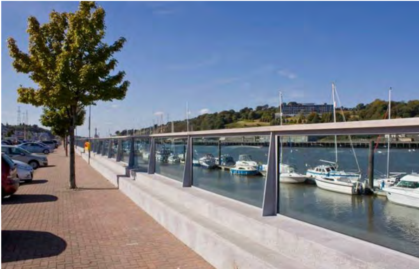
Flood protection barrier of glazed panels at Waterford, Ireland
