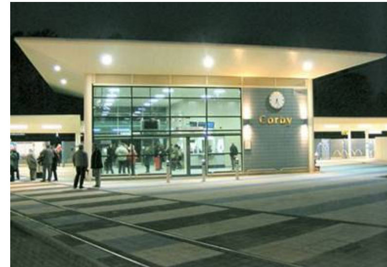
Figure 5.14 – Recently completed Corby Railway Station
