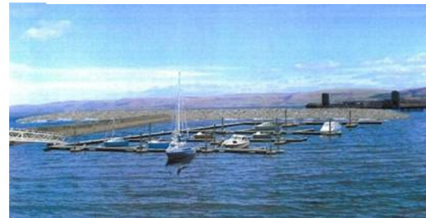
Figure 3.13 – West Pier demolished
