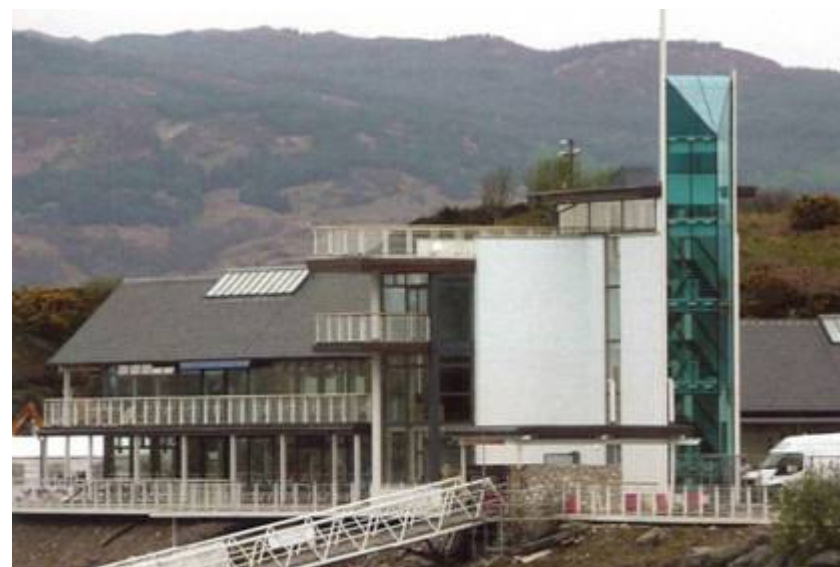
Figure 5.5 – New marina facilities building, Portavadie Marina
