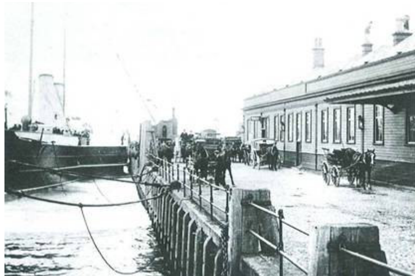
Figure 5.19 – Historical photograph of Stranraer Harbour Station
