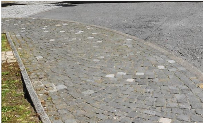
Some examples of natural stone setts near to the Town Hall and Library
