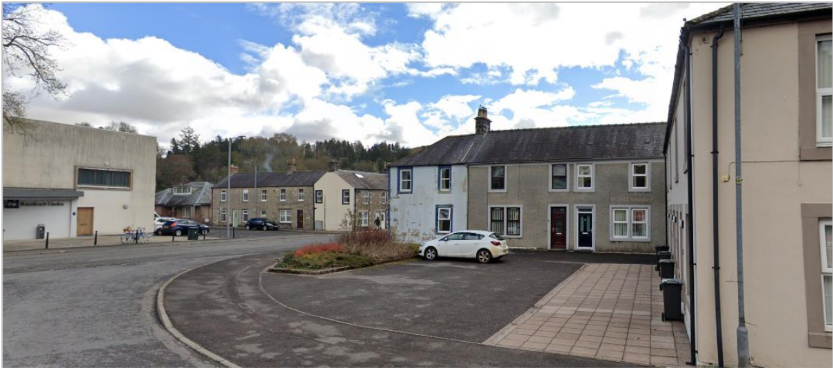
South-east side of Buccleuch Square with Thomas Telford Road passing through
