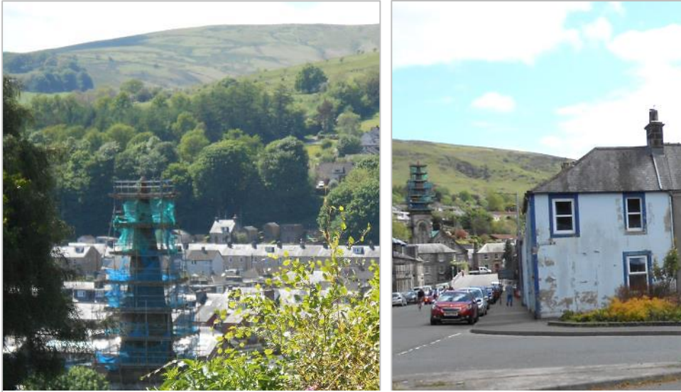
Scaffolded Erskine Church spire is prominent in a number of views.
