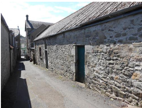
Former bakery building in vernacular, rubble wall behind the High Street on Well Close possibly from 18 th century
