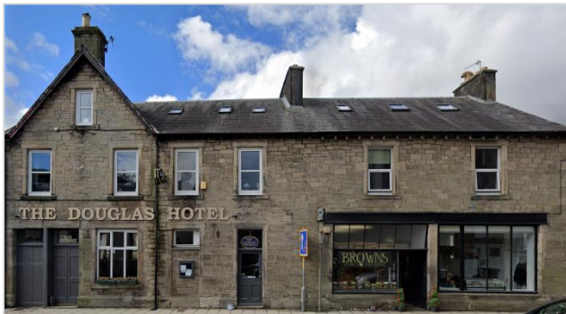
The Douglas Hotel – unlisted elegant town building with advanced gable at eastern end built from random coursed, cut Whita sandstone with simple window margins in same stone. One side a hotel and the other with an interesting traditional shop at ground floor.
