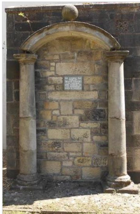
The Telford Arch in Parliament Square built by mason, architect and engineer Thomas Telford for the King's Arms Inn and brought here.
