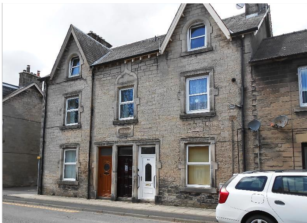
Below: 2½ storey pair on Henry Street with front facing gables in Whita stone including an 1897 date stone
