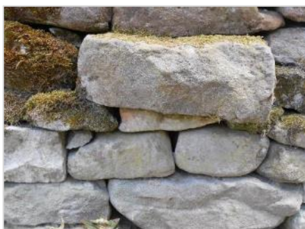
Left: dry stone wall built from Whita stone
