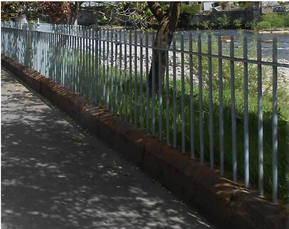
Linear railings on a sandstone base along the River Esk, Elizabeth Street
