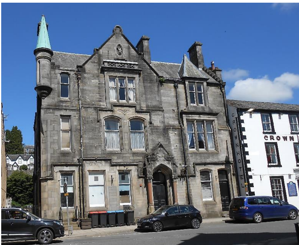
Above: C Listed RBS building on High Street with some Scots baronial detail
