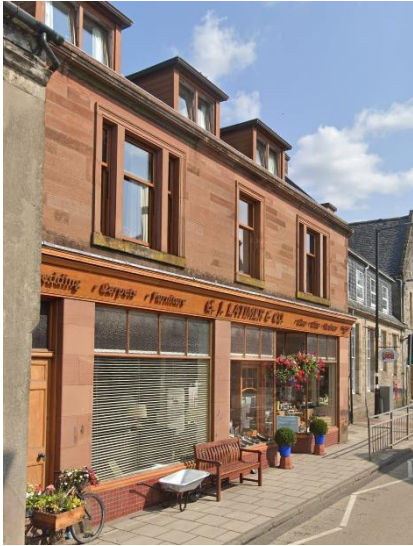
Latimers, High Street unlisted 1926 red ashlar sandstone shop. Very distinctive among the pale sandstone buildings and a key local business.
