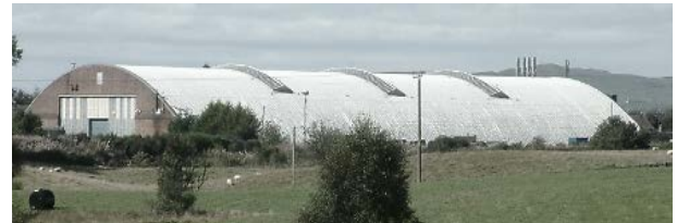
Former plane hangar at Heathhall
