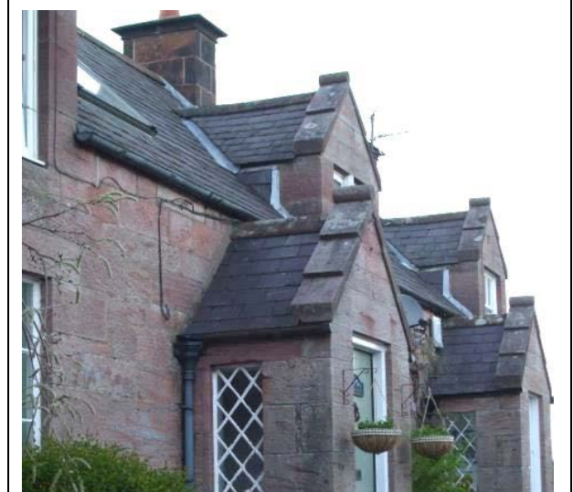
Proportionate gabled dormers on stone cottages
