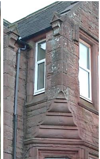
Patterns of slatework found in region. Sandstone drip moulds over gate lodge door; unusual corbelling detail on corner of sandstone house.
