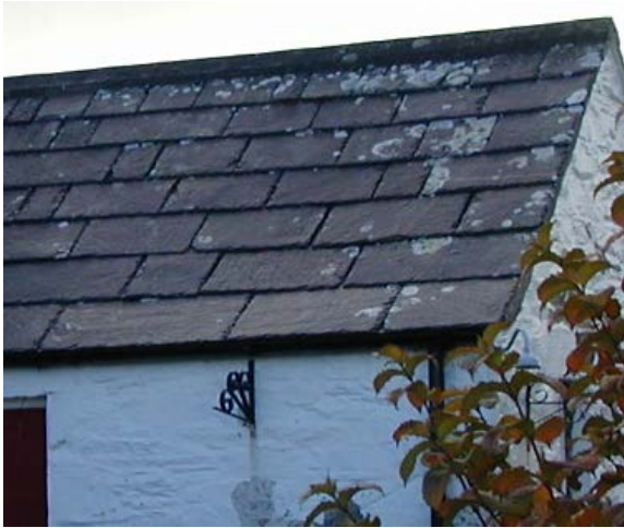
Graded Lancashire slate roof
