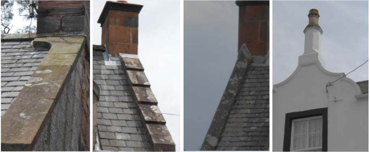
Examples of varied roof line details: a selection of skewstones – stepped, shaped, interlocking and plain; a shaped gable stack; and decorative skewputts and finial
