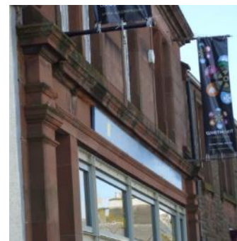
Early 20 th century commercial building in Whithorn, which differs from its neighbours due to use of ashlar sandstone and classical details
