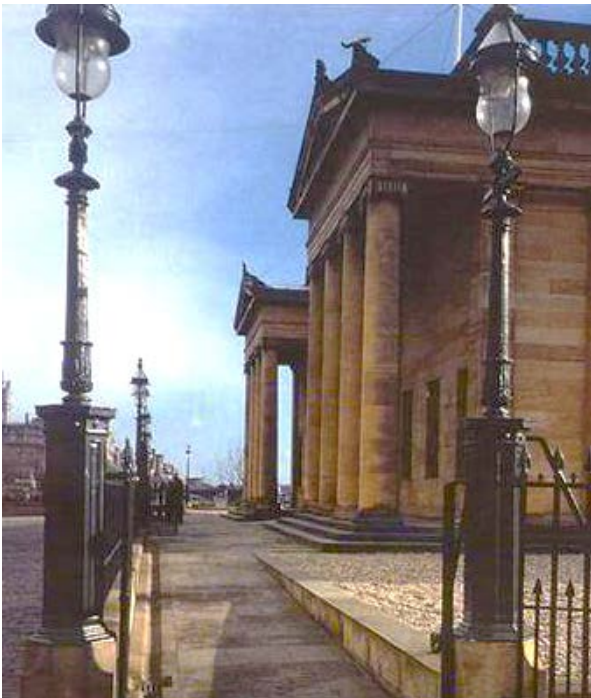
Access ramp to National Gallery of Scotland
