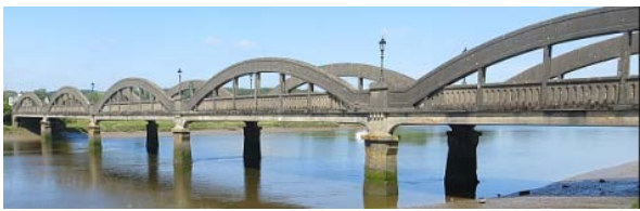
Early 20 th century reinforced concrete and steel bridge, Kirkcudbright
