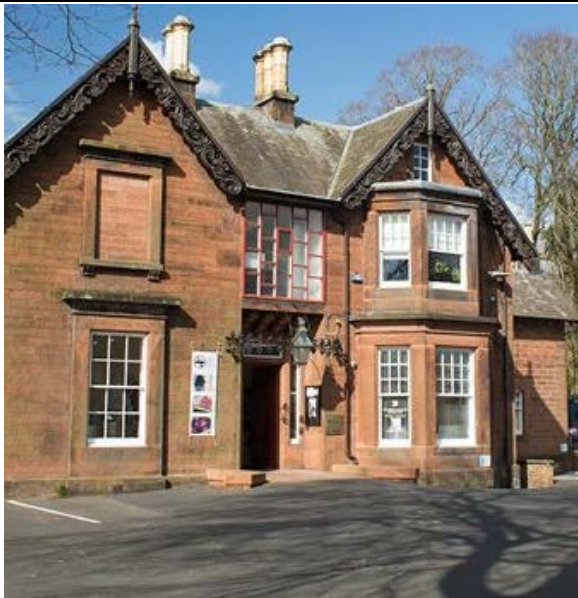
Gracefield Art Gallery - the slope on the tarmac apron was raised to the level of the top step.
