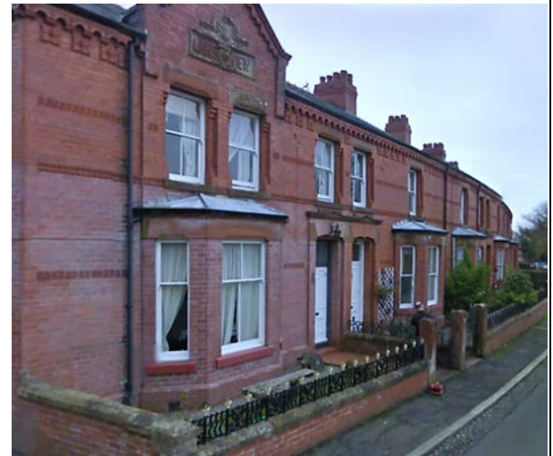
Lakeview Terrace, Powfoot - a continuous brick façade with string course and cornice; regular bay windows and chimneys and front facing gable 'end stops'.
