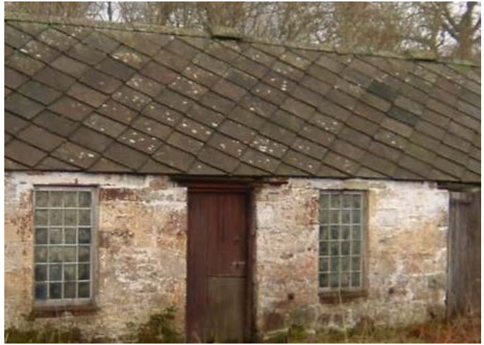
Sandstone flagged roof
