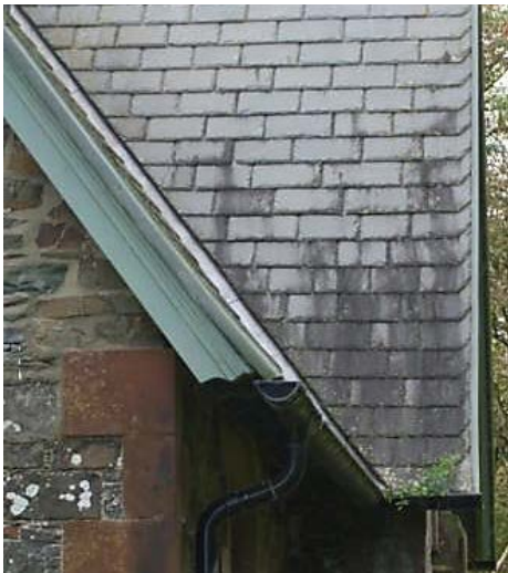
Lodge with overhanging slate roof, angle cut tiles and verge board; decorative slate work and example of 'double lap open tally' slating in Nithsdale.
