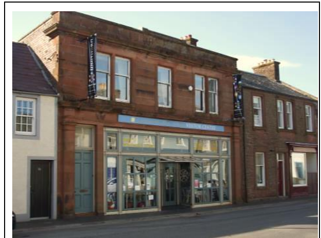
Early 20 th century commercial building in Whithorn, which differs from its neighbours due to use of ashlar sandstone and classical details
