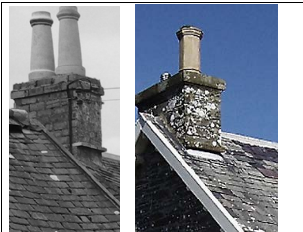
Chimneys with thackstones: evidence of earlier thatching
