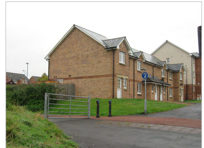
Footpath links at the Marchfield development
