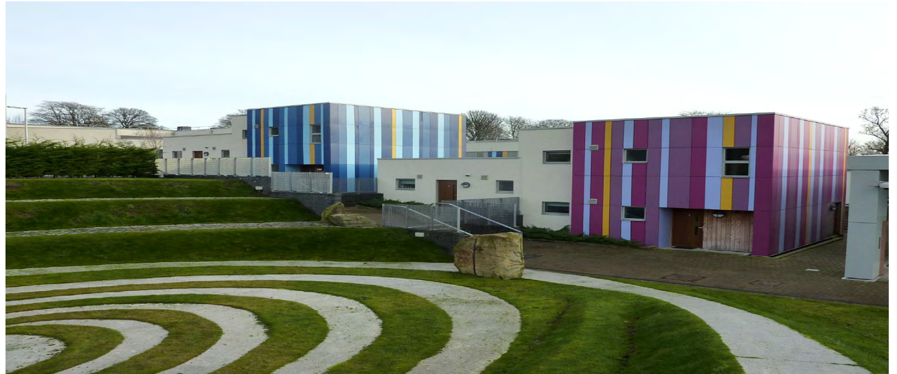
Midpark Hospital, Dumfries which uses the sloping site to its advantage
