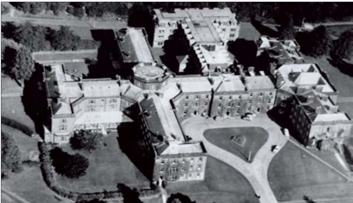
Figure 3.1: Above is a 1950s aerial view of Crichton Hall. Built in 1839, the Hall was the first part of Crichton Royal Institution. Architect William Burn's intended design was two linked Greek crosses each with central octagonal stair turrets. However, only one cross was completed.
