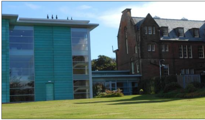
Figure 5.6: Johnston House and its dramatic extension which uses a very contrasting form and materials palette. It joins with the 19 th century Sydney Mitchell building using a low, glazed link.
