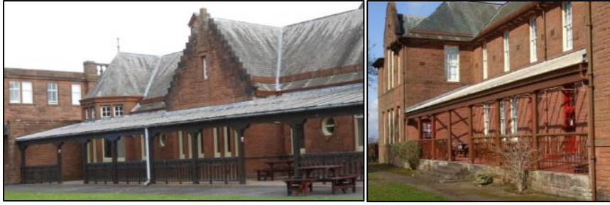
Figure 3.2: From the beginning, doctors at Crichton Royal Institution wanted patients to benefit from the outdoors. Open glazed arcades were included on the upper floors of Crichton Hall; although glazed in subsequent years. Many late 19 th and early 20 th century villas had west facing verandas. Criffel View and Monreith House are shown.
