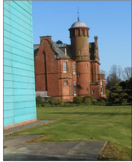
Figure 5.6: Johnston House and its dramatic extension which uses a very contrasting form and materials palette. It joins with the 19 th century Sydney Mitchell building using a low, glazed link.
