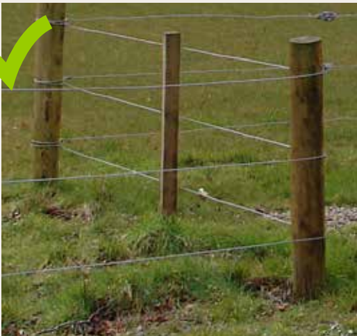
simple unobtrusive post and wire fencing
