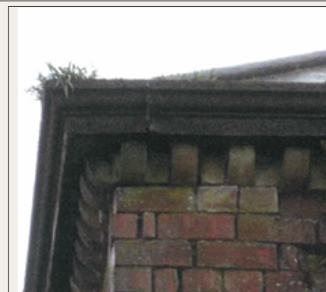
Kelton stables: use of brick with feature eaves
