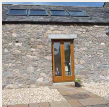
Jordieland; light grey pink field stone forms rubble wall, note new concrete lintol above door opening; no ashlar quoins
