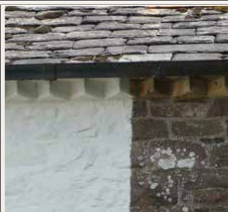
Boatcroft: painted finish over dark grey/red stone brick decorative feature below eaves
