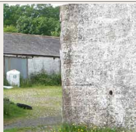
Thornhill; residual limewash on red sandstone
