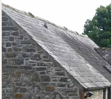
plain eaves & verge detail with no gutter
