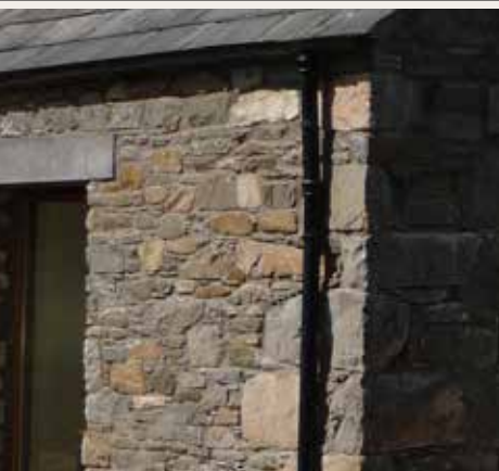
Jordieland; light grey pink field stone forms rubble wall, note new concrete lintol above door opening; no ashlar quoins
