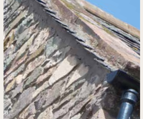
slates extend behind cope
