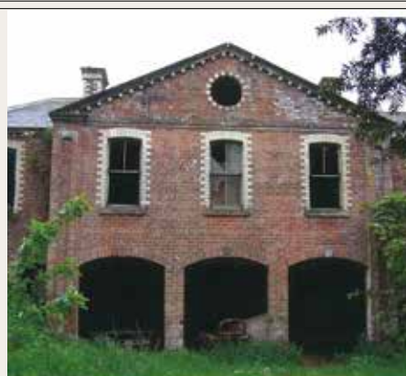
Kelton stables: use of brick with feature bricks at window surrounds
