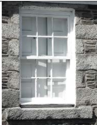
6 over 6 pane sliding sash and case window with operational shutters
