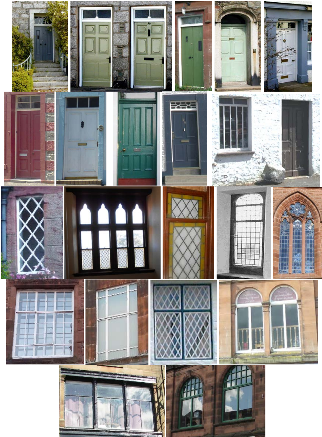
WINDOWS AND DOORS IN LISTED BUILDINGS AND CONSERVATION AREAS
